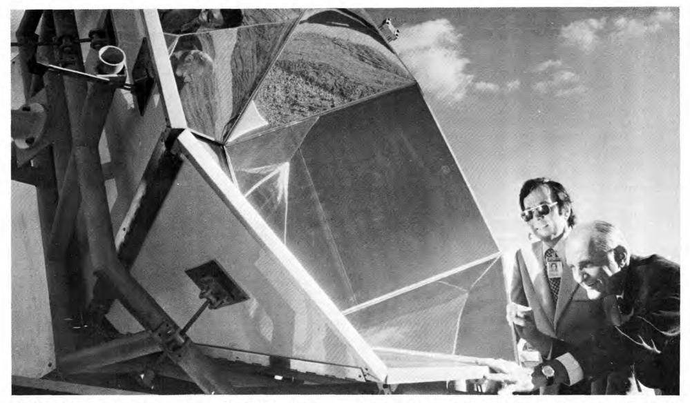
ON THE SUNNY SIDE — Albuquerque Journal for Jan. 23 carried Labs release on Sandia's solar energy pilot project to provide electricity, space heating, air conditioning, and hot water for Bldg. 832. About 10,000 square feet of solar collectors will be needed to generate needed energy. Recent AEC committment of
